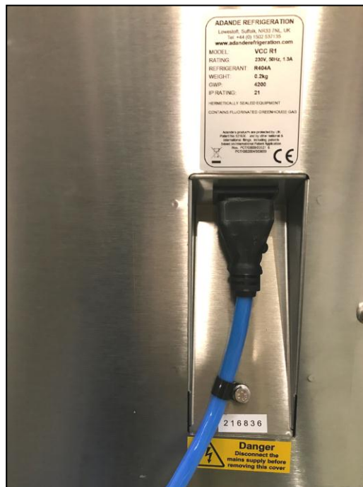
Figure 3: Mains connection point
